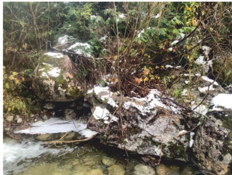
Upstream left bank riprap
