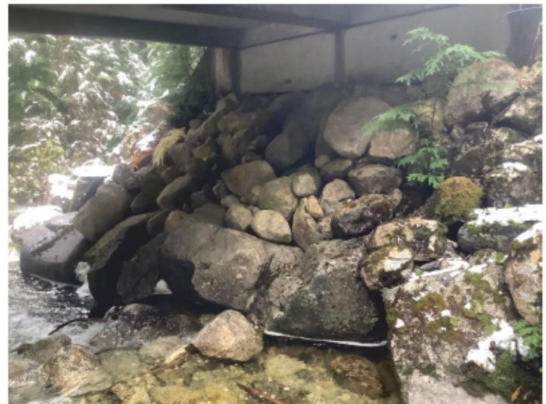
Right Bank Abutment when facing downstream
