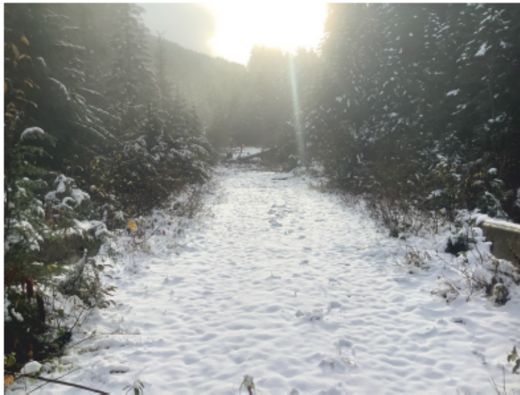
Approach from bridge deck of Right bank approach when facing downstream
