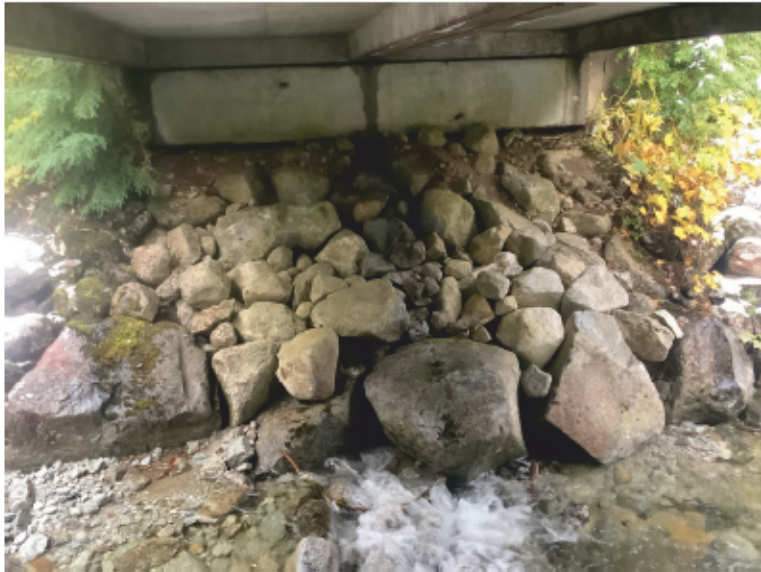
Left Bank Abutment when facing downstream
